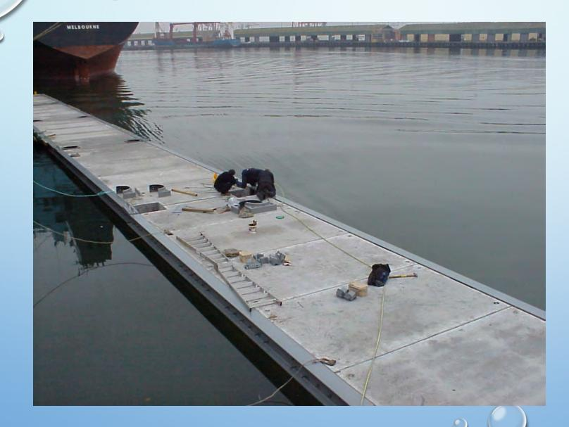
Bellingham Marine made a name with the **Unifloat** system of floating pontoons – a system of custom-made elements, each suited to the specific location and its conditions.
